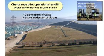
Resistivity well suited for monitoring bio-degradation process
